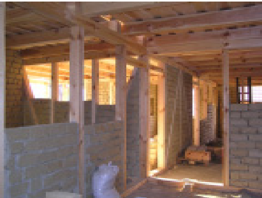
Fig. C5 – vista interior I.
