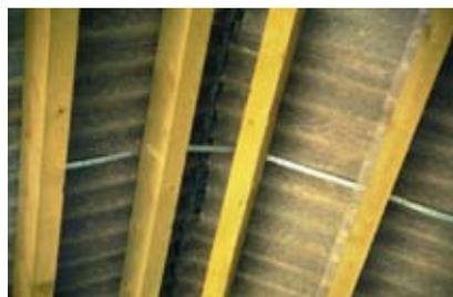
Figure 21. Diagonal truss of corner module
