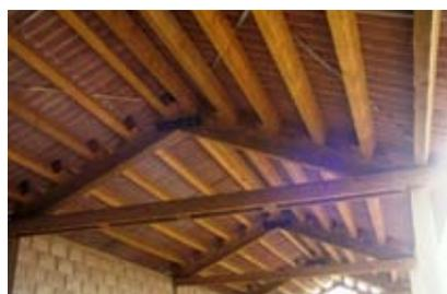
Figure 19. Standard module and truss with bracing
