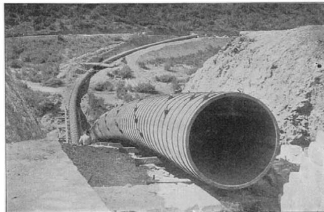
FIG. 158. Redwood Stavepipe (36 inch) Crossing Warm Springs Cañon, near Redlands, California.
