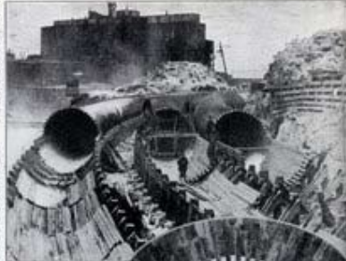
THREE HUGE PIPES
