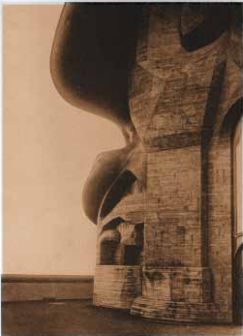
Rudolf Steiner's First Goshuarum Exterior 0025 The finished First Goshuarum circa 1921. The north wing of the east portal.
