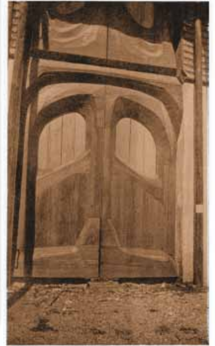
Rudolf Steiner's First Goshuarum Exterior 0019 The finished First Goshuarum circa 1921. The lower entrance of the east portal.
